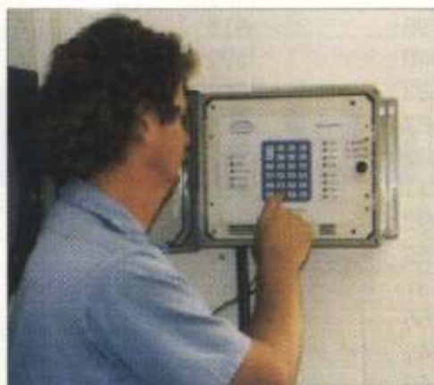
DialLog Plus alarm monitoring and automatic notification units can monitor up to eight alarms. Other DialLog units can monitor up to 40.
